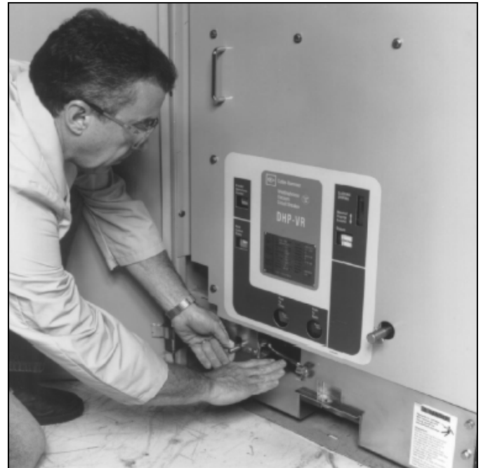
Figure 4-12 Final Engagement of 7.5 or 15 kV Secondary Contact
