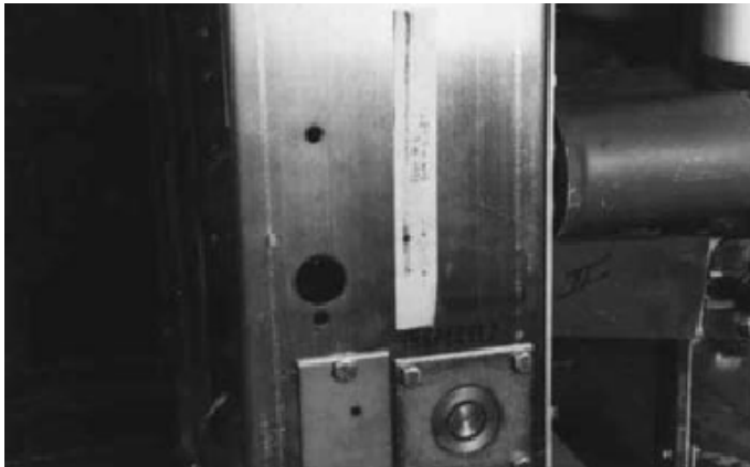
Figure 6-18 Place Tape on Right Side Panel of Breaker
