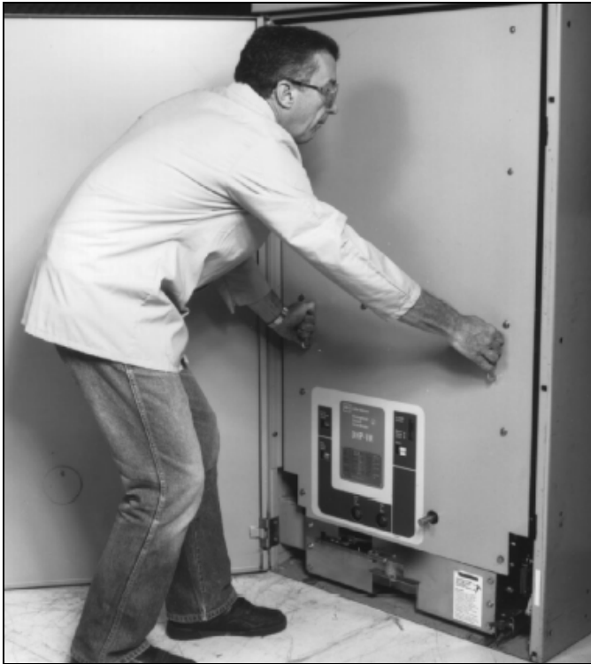
Figure 4-10 Positioning of 7.5 or 15 kV DHP-VR Breaker
