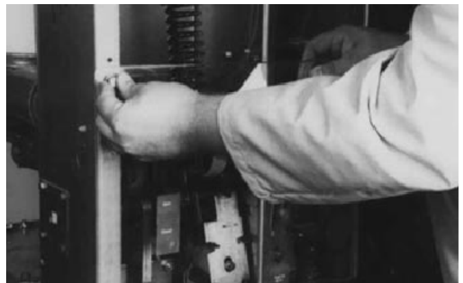
Figure 6-10 Attaching CloSure™ Test Tool at Hole "A"
