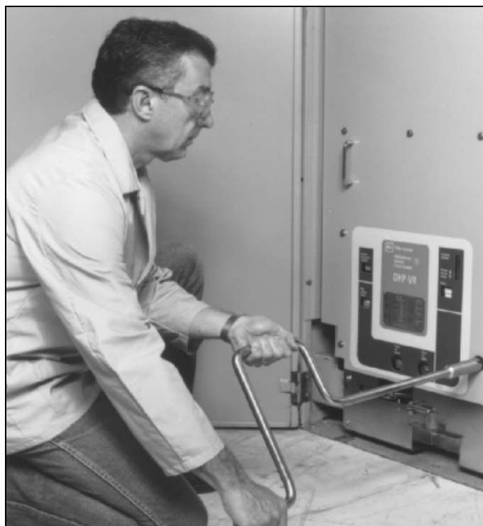
Figure 4-14 Levering 7.5 or 15 kV Breaker to Connected Position
