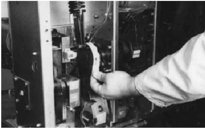
Figure 6-17 Remove Marked Masking Tape from Cam
