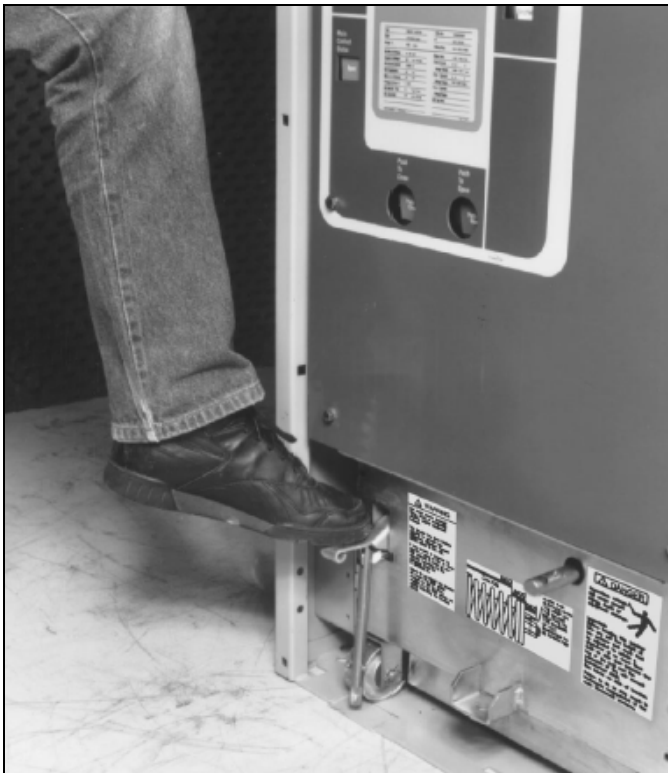
Figure 4-11 Final Engagement of 5 kV Secondary Contact
