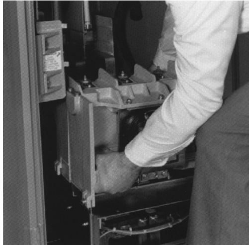
Figure 13 Removing the Contactor
