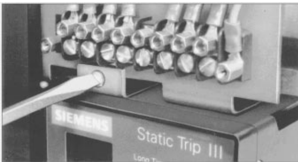
3.) Secure the trip unit with a single (1) #6-32 mounting screw.
