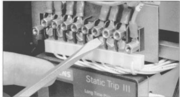
4.) Align the terminal block fanning strip with the terminal block secure it with the eight (8) #6 - 32 slotted head screws
