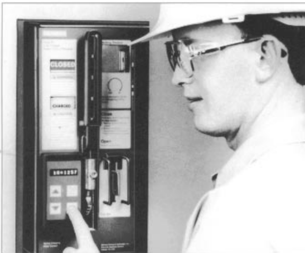
BDU Mounted on Type RL Circuit Breaker
