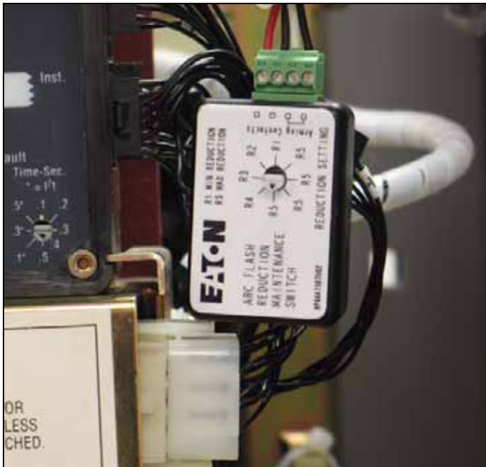
Figure 11. RSM Connected to the Trip Unit and External Harness.
