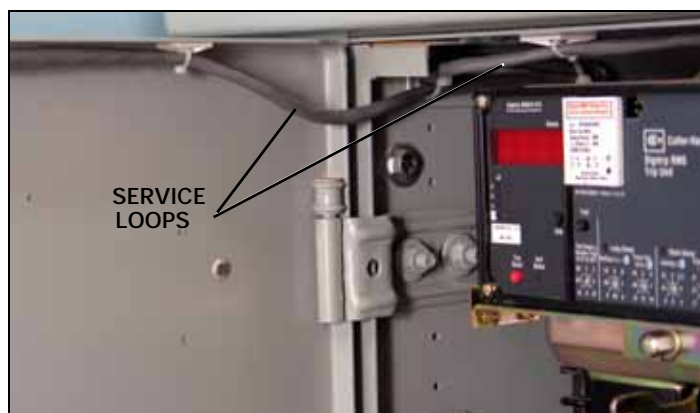
Figure 27. Routing of the Mode Selector Switch Harness and the Service Loop.
