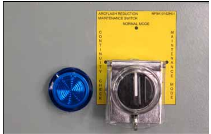
Figure 22. Indicator Light Installed on the Mounting Surface.
