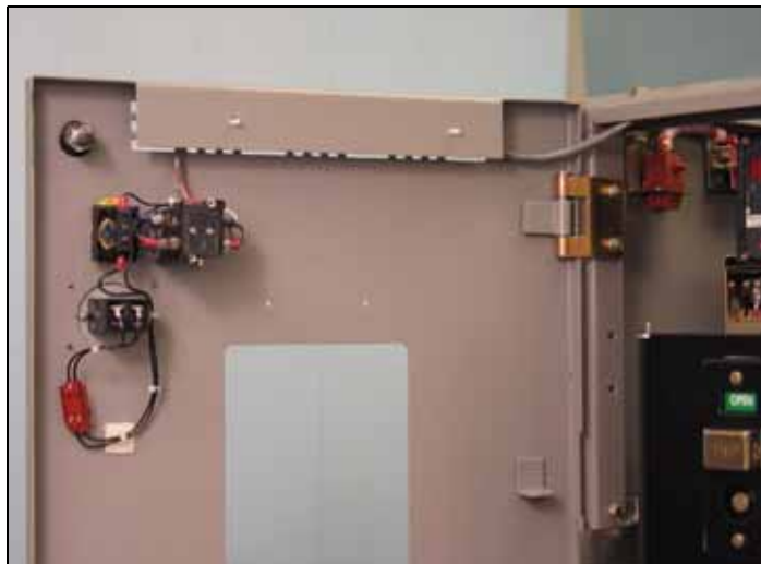
Figure 25. Overview: Final Wiring of the RSM, Mode Selector Switch, Indicator Light, and Battery Holder.
