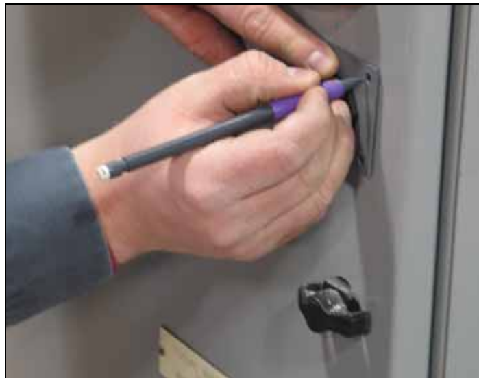
Figure 17. Marking the Battery Holder Mounting Holes.
