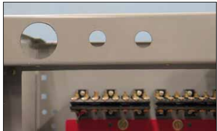
Figure 13. Alternate Mounting Location on Certain DS Applications.
