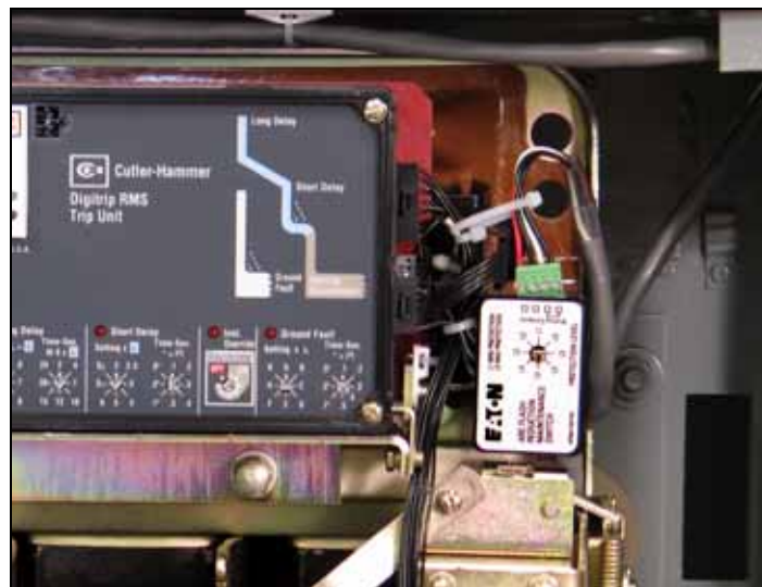
Figure 8. Overview: Arcflash Reduction Maintenance Switch Components Installed on a Non-DS Breaker.
