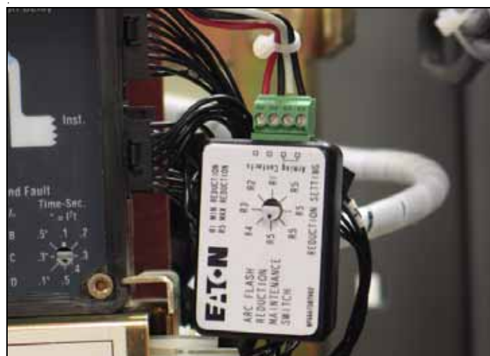
Figure 28. Mode Selector Switch Harness Connected to the RSM.
