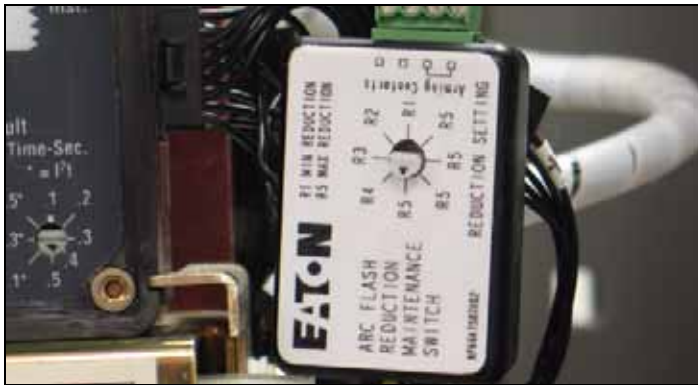
Figure 30. Selecting the RSM Reduction Setting. R1 = Min. Reduction, R5 = Max. Reduction.
