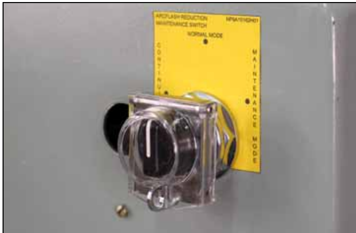
Figure 20. Mode Selection Switch and LOTO Installed on the Mounting Surface.
