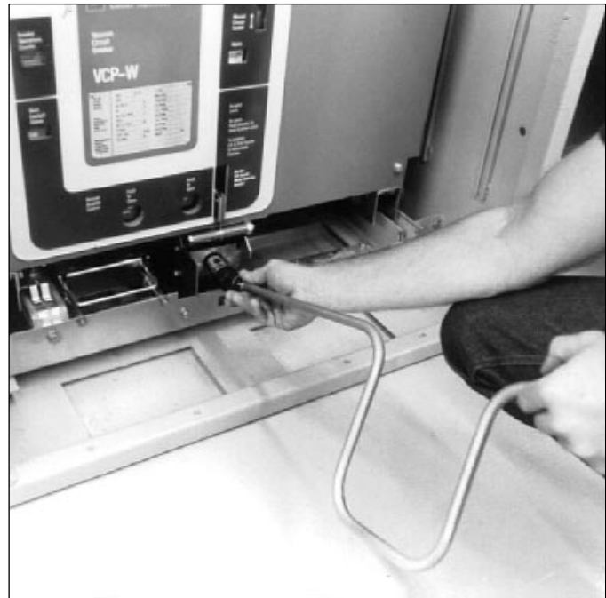
Figure 4-6 Engaging Levering-In Crank
