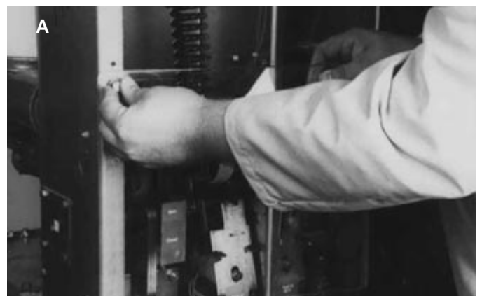
Figure 6-9 Attaching CloSure™ Test Tool at Hole “A”
