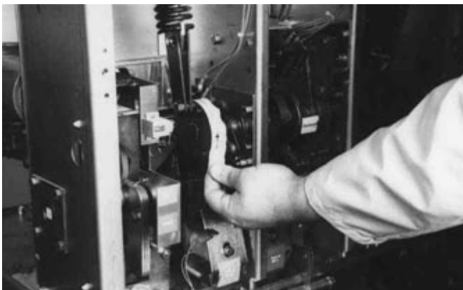
Figure 6-16 Remove Marked Masking Tape from Cam
